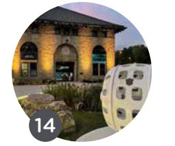
14 Niagara Parks Power Station + Tunnel
